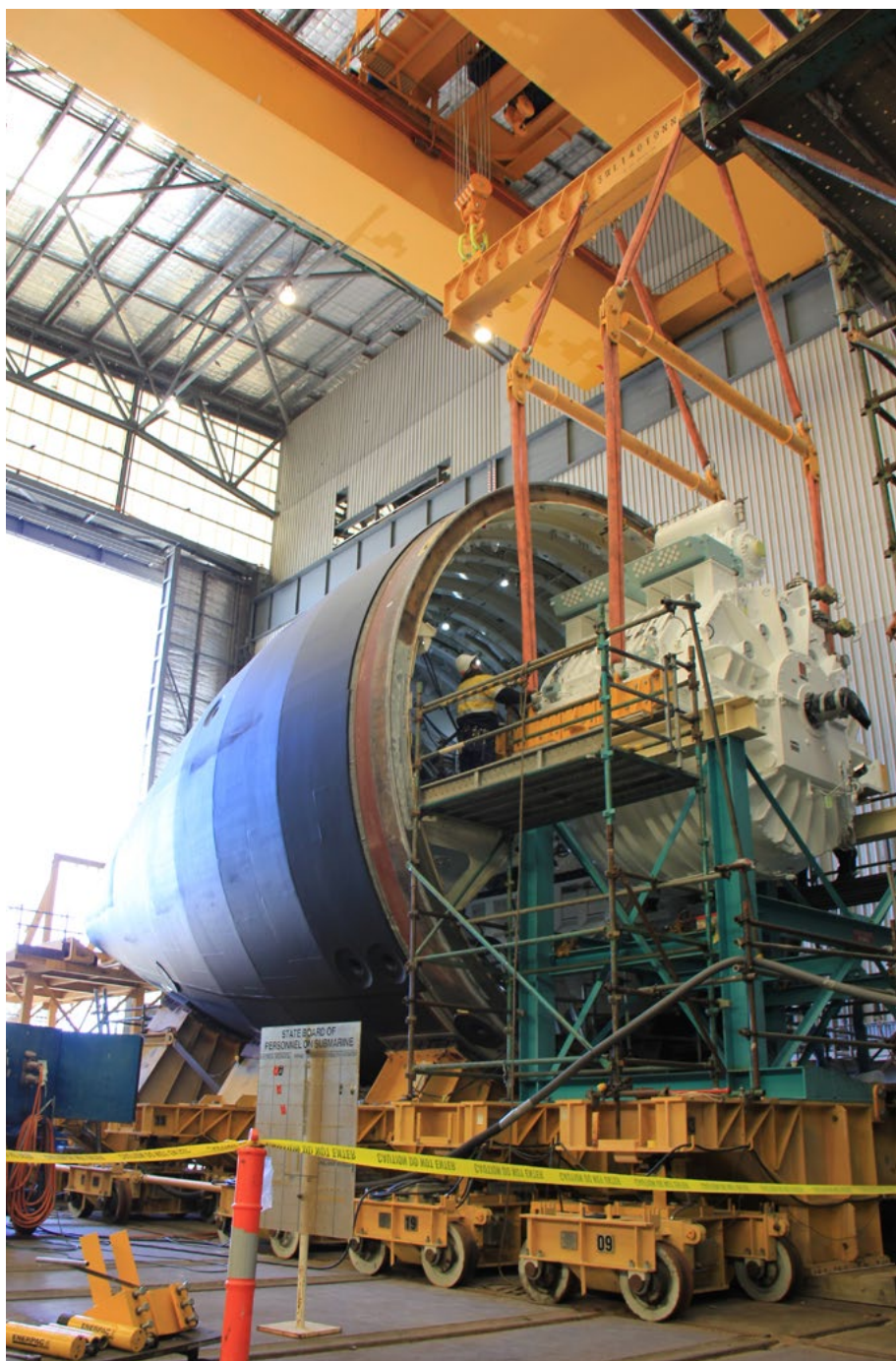
Cutting the hull allows easier access to major components such as the diesel engines and, as seen here, the electric motor. (Photo courtesy ASC).
