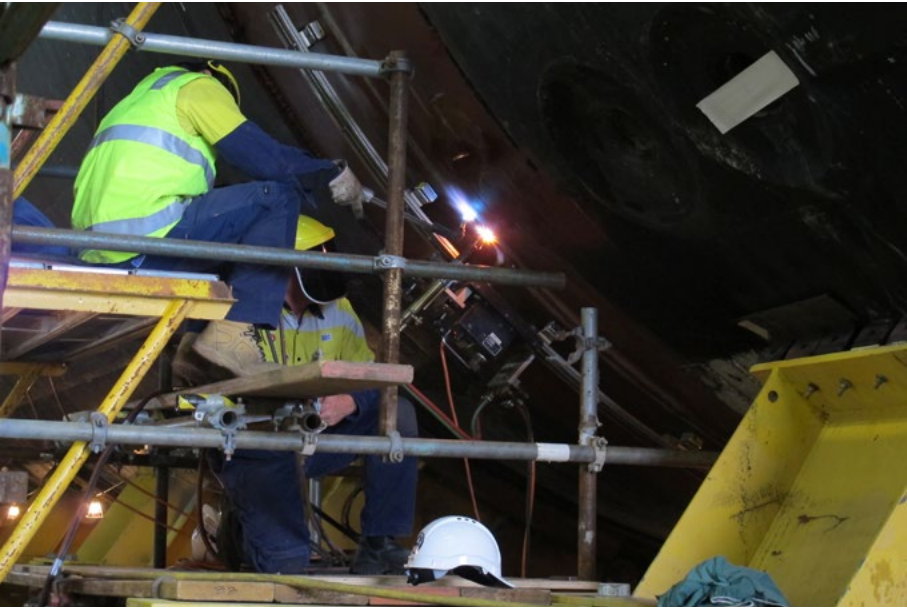
Although controversial at one time, it is now standard practice at ASC to cut the hull of a submarine undergoing a full-cycle docking. (Photo courtesy ASC).
